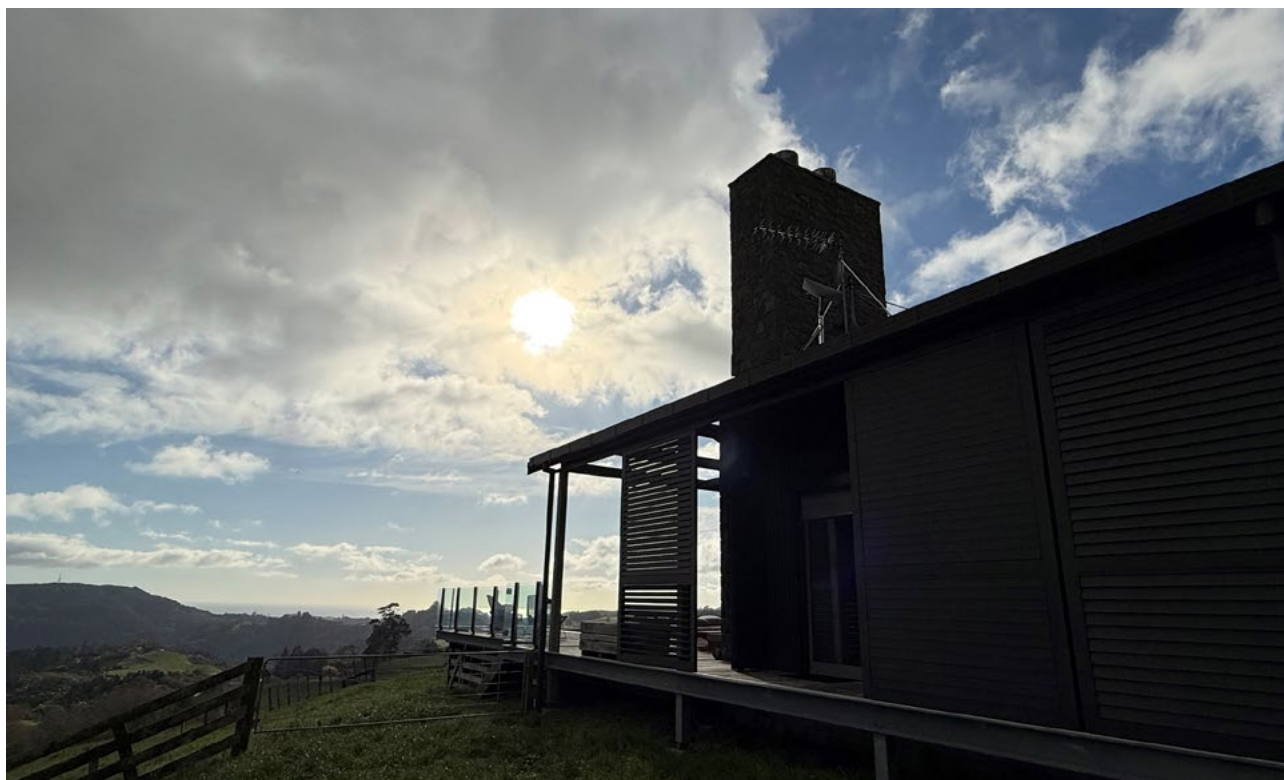
Top: Starlink Dish on roof.
